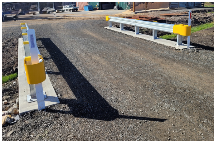
Upgraded Maintenance Cross over at Yarram site
